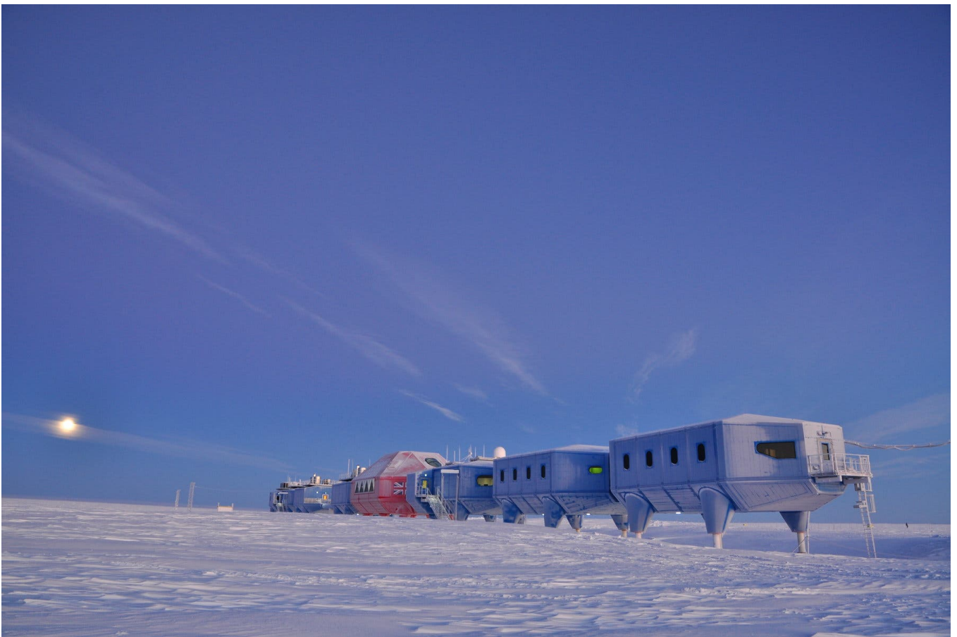
Britain's Halley VI, designed by Broughton Architects, sits on hydraulic stilts and on skis. Antony Dubber
